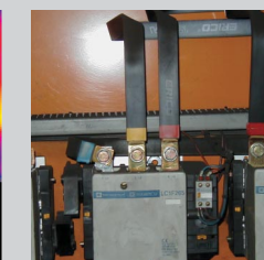
Electrical: Termination problem on yellow phase
