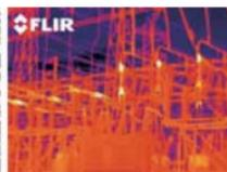
**Substation** - A wide view of a substation can quickly show areas where unwanted high resistance connections exist. Electrical current passing through a resistive connection produces heat; electrical systems get hot when connections loosen or corrode and power is not properly transmitted — no other predictive maintenance technology is as effective for electrical inspections as IR thermography.
