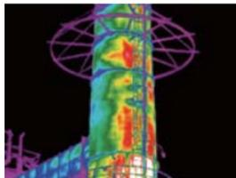
**Refractory lined equipment** - Furnace refractory breakdown a crude heater stack is clearly shown in this thermal image. If it is unchecked, the condition would accelerate and cause metal degradation and catastrophic failure.
