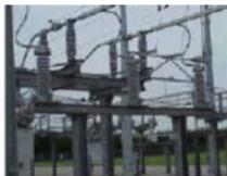
**Regular IR Scans Keep the Lights On** - Electric companies must have reliable power lines to provide their customers with the service they expect and deserve. Unfortunately, when lightning arresters fail, the whole system hangs in the balance. Regular inspections can help prevent power outages by detecting bad lightning arresters in substations and faults in distribution lines.
