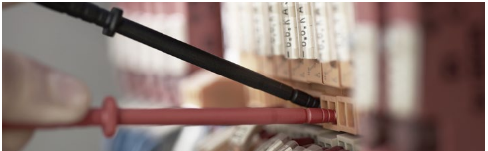
Measurements in fuse boxes and switch cabinets
