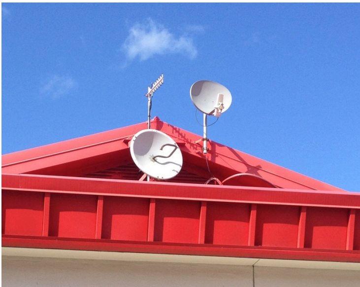
Figure 5: Yagi used as a donor antenna
