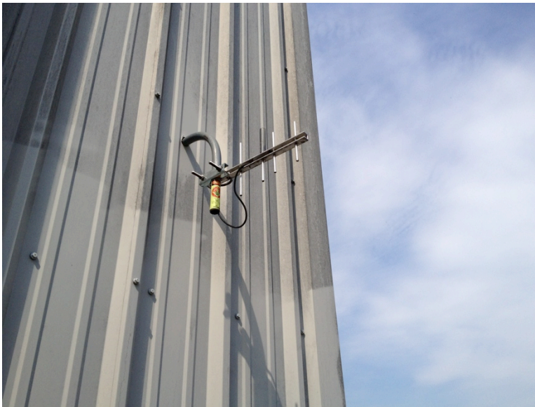
Figure 8: Small yagi on a metal building – possible BDA installation
