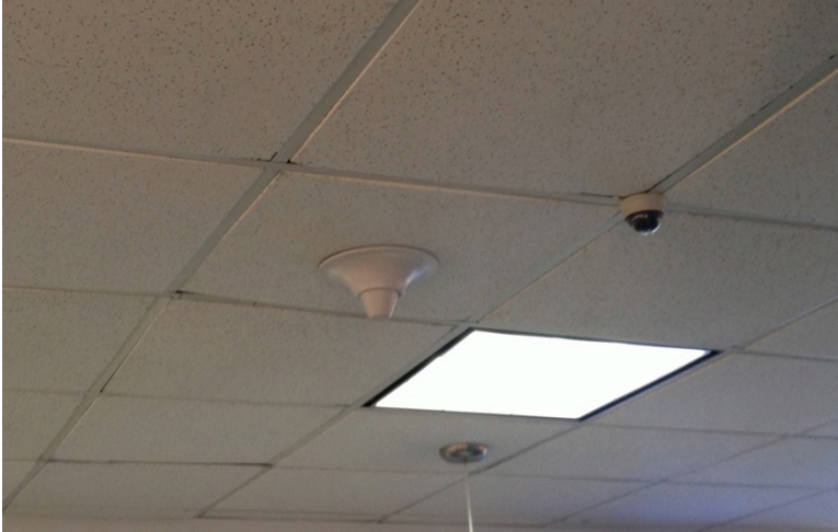
Figure 11: Ceiling-mounted dome antenna used as a serving antenna
