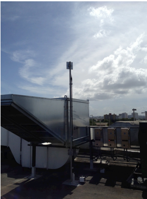
Figure 7: Roof-mounted panel antenna used as a donor antenna
