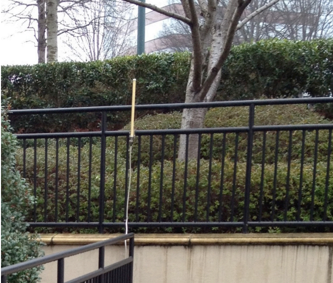
Figure 6: Omnidirectional vertical used as a donor antenna
