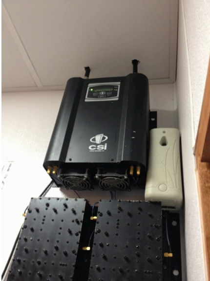
Figure 13: Bidirectional amplifier
