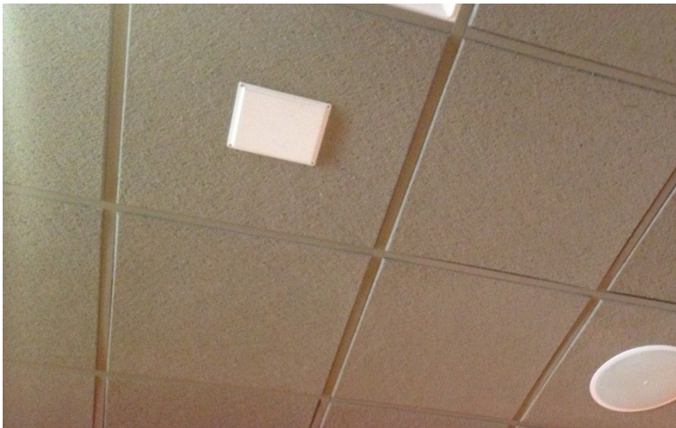
Figure 10: Ceiling-mounted panel antenna used as serving antenna
