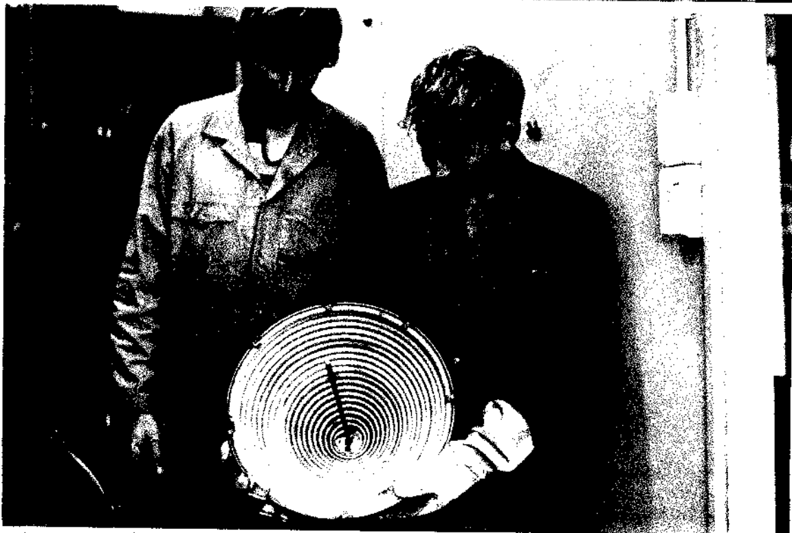
Figure 59(a) Winding a Mark III absorber
