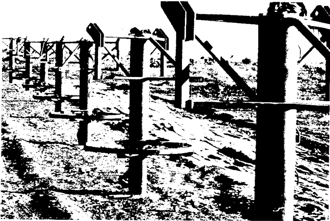
Figure 65 - Pedestal supports set in the ground, preparatory to mounting dishes
