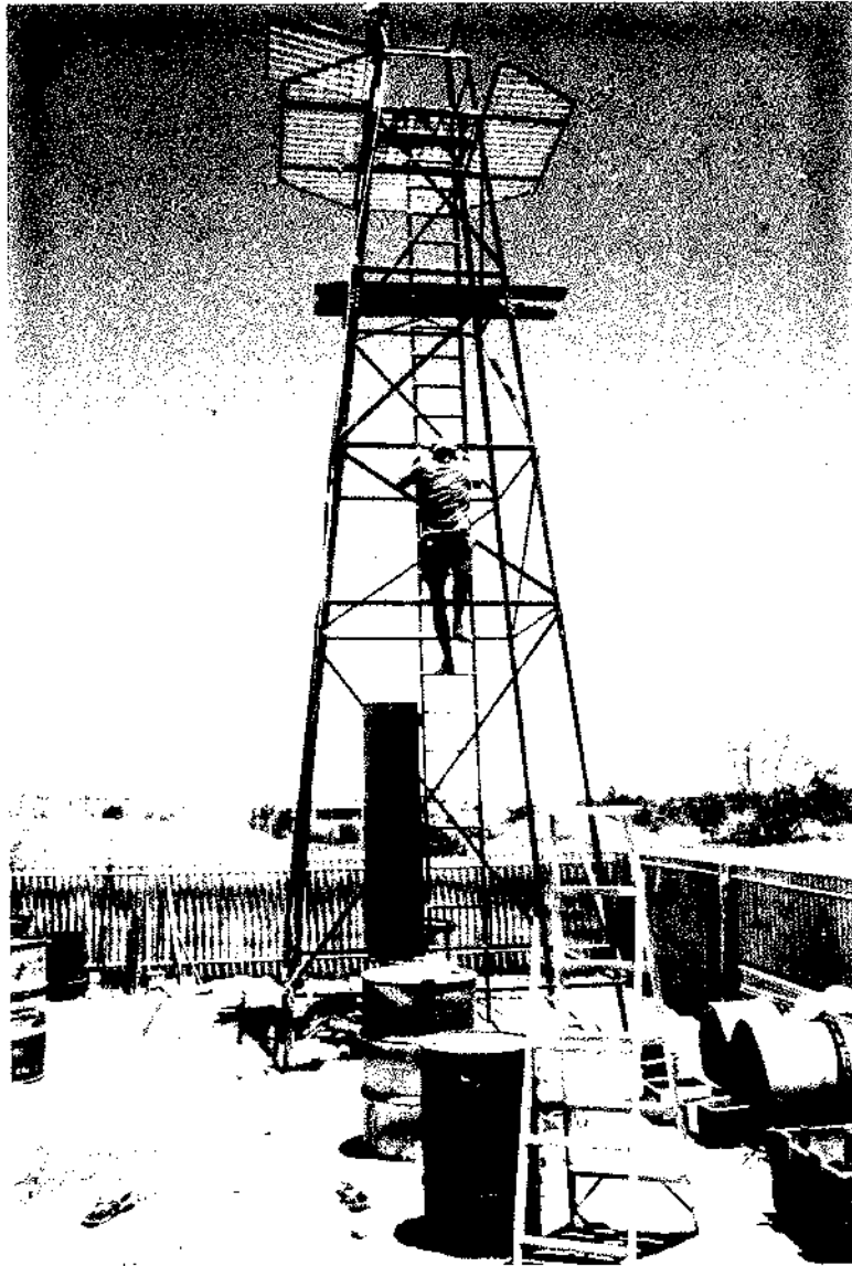
Figure 52 - Seven metre Tower for mounting sun and wind monitoring instruments (December 1979) in the yard of the White Cliffs Hotel (Subsequently relocated at the Station site
